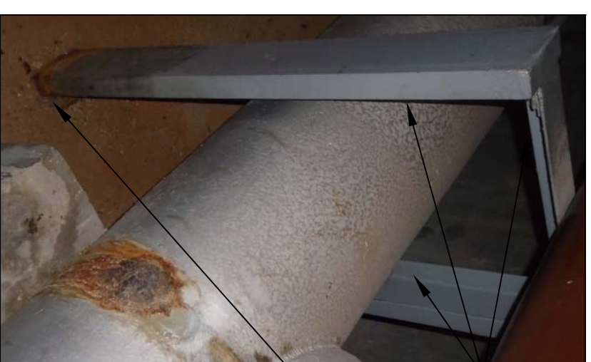
TYPICAL FLOOR FRAME SUPPORT
